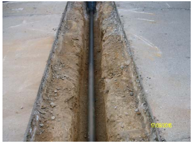
66. Tram 4: Rasa creuament c.Jordi Girona (AGBAR)
